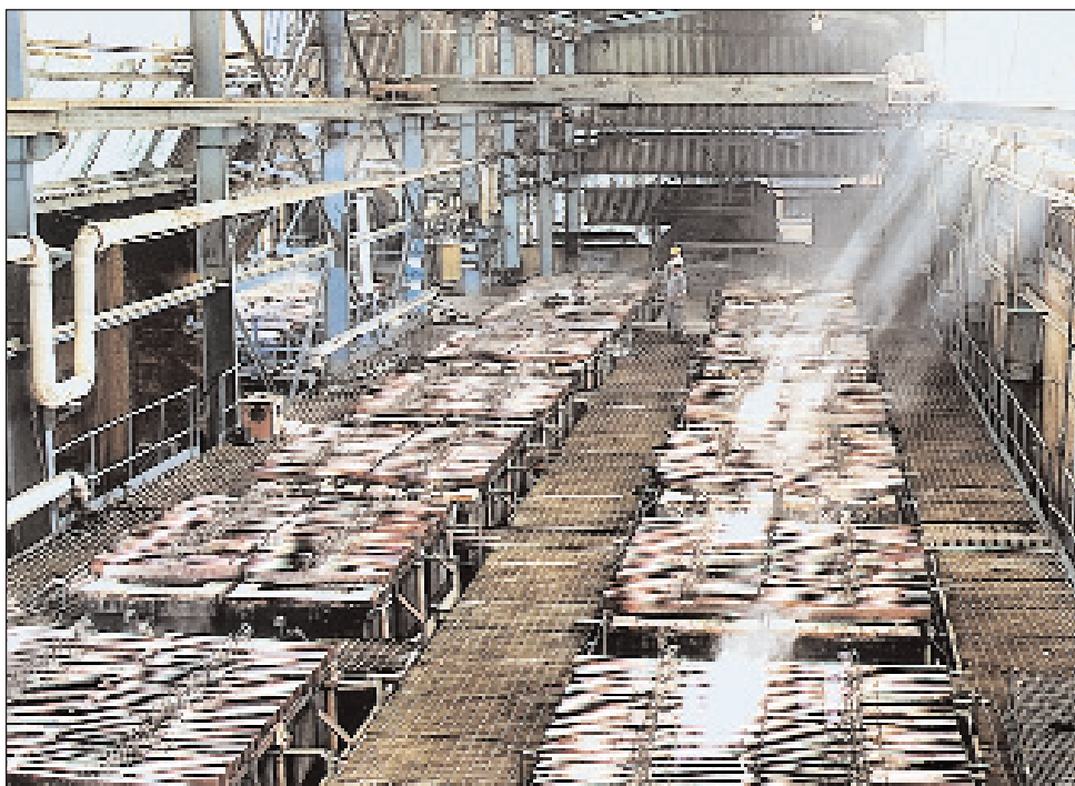
Electroplating Section of EMD Plant Dongri Buzurg Mine
