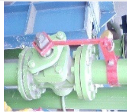
Energy Isolation Arrangement for Valves
