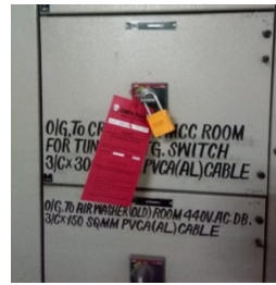
Electrical Energy Isolation Arrangement
