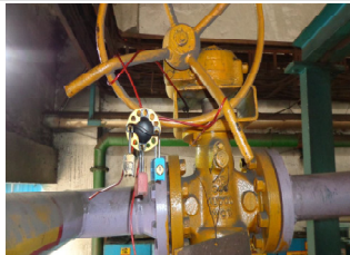
Energy Isolation Arrangement for Valves
