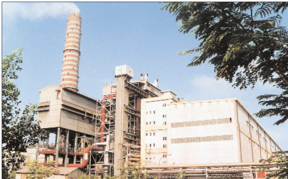
Visakhapatnam Steel Plant — Thermal Power Plant
