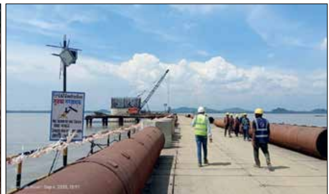
Palasbari – Sualkuchi River Bridge
