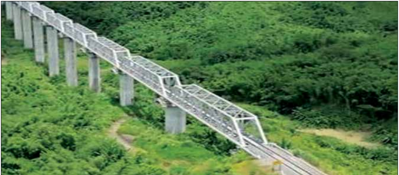
Bairabi-Sairang railway project in Mizoram.
