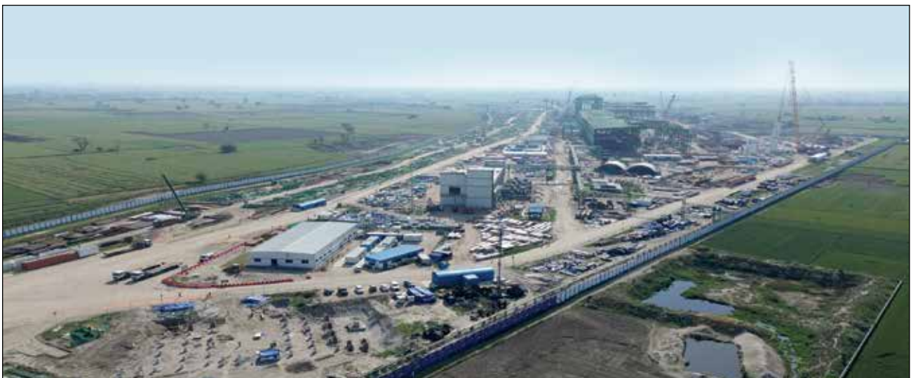
Aerial View of steelmaking facility in Ludhiana
