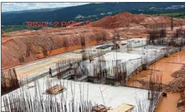
Meghalaya New Secretariat Building
