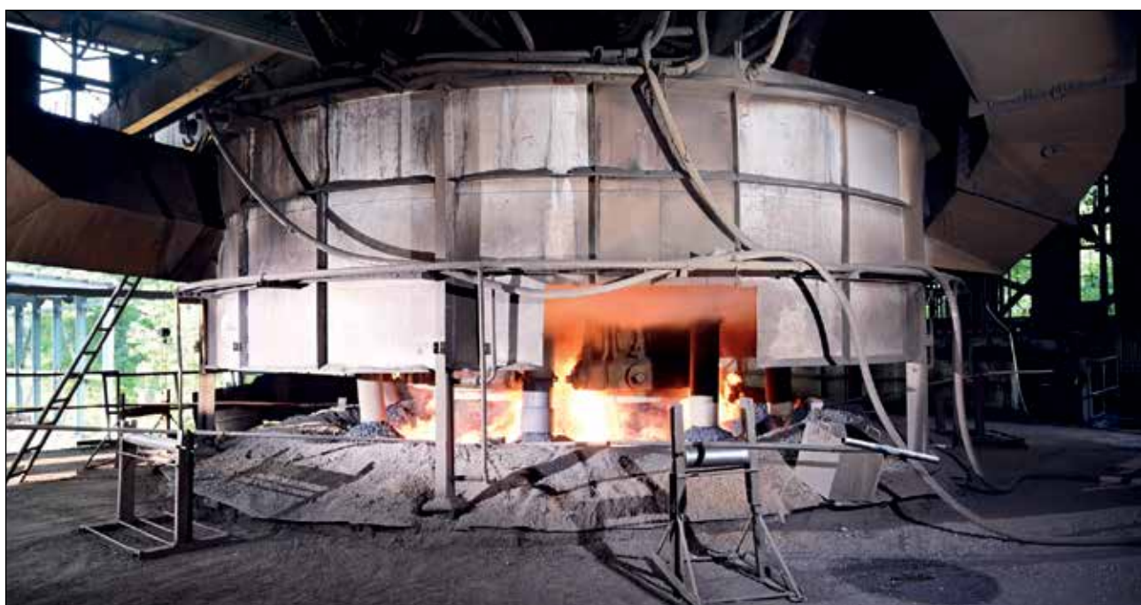
FMP Furnace at Balaghat Mine, MOIL
