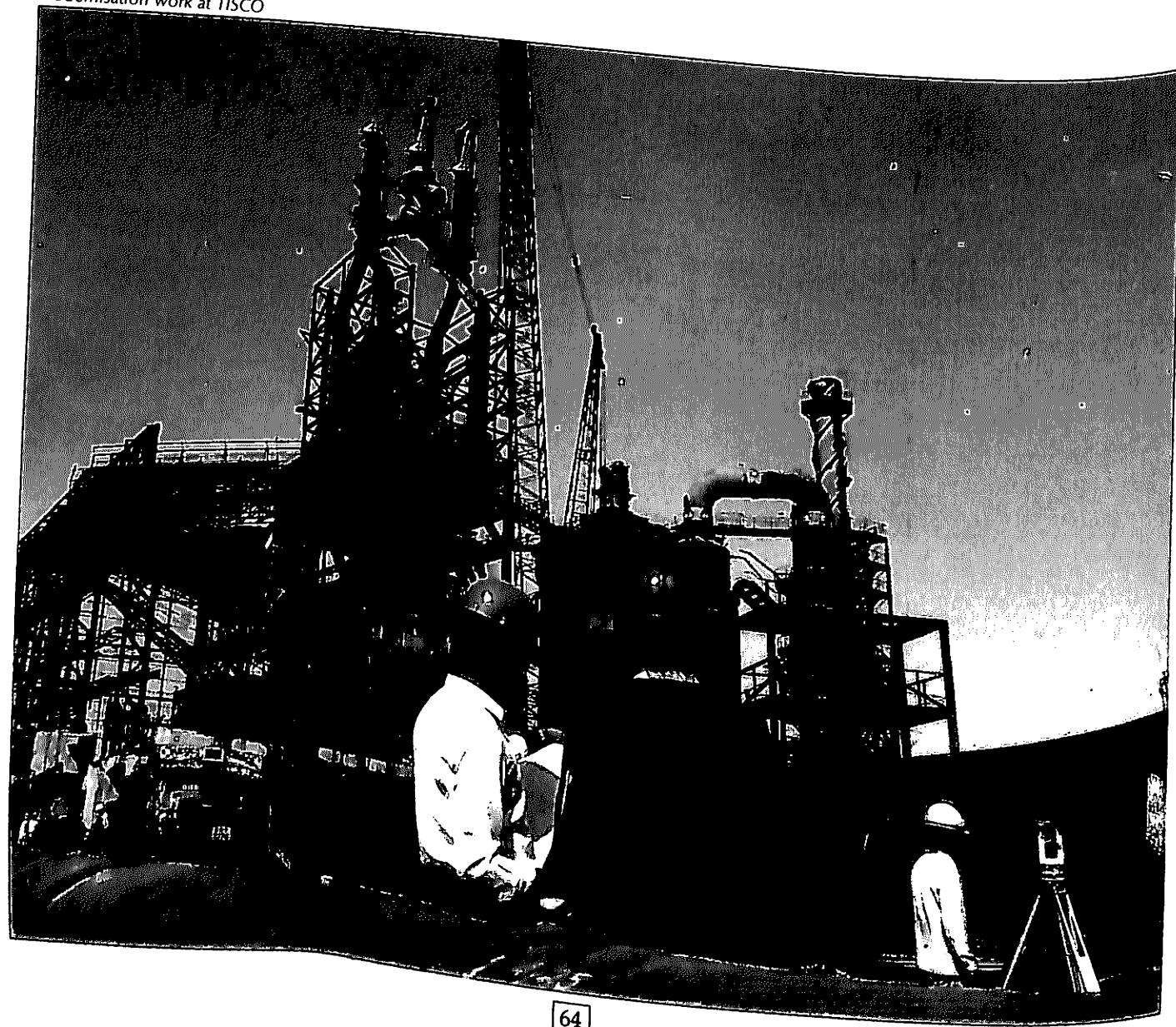
Modernisation work at TISCO
