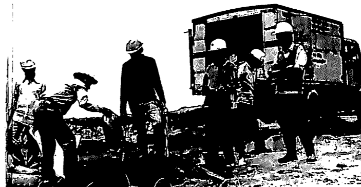
Blasting operations are in progress at Bailadila deposit-5
